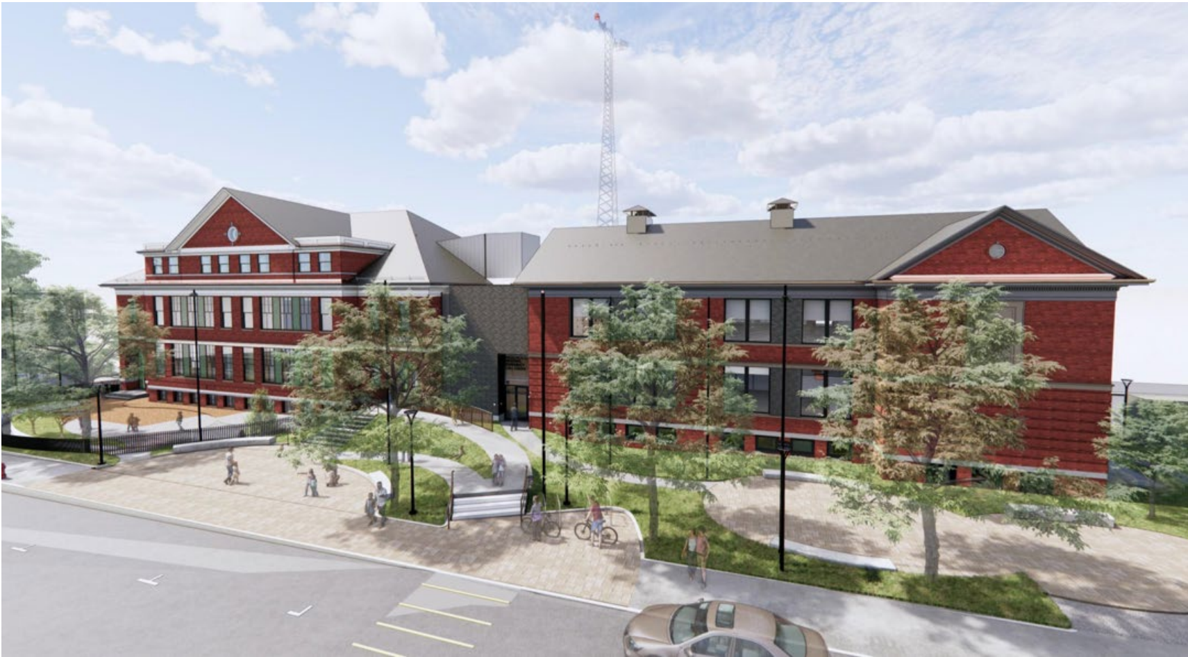
Figure 2: DPCD is leading the McKinley School renovation, into a 911 Call Center, Early Childhood Center, and municipal offices. Construction is scheduled to begin in 2026
