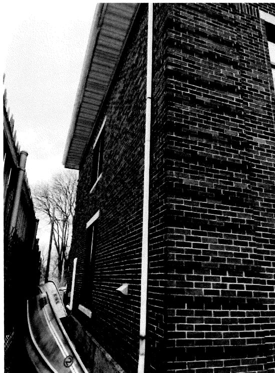
Building Rear View (West side)
