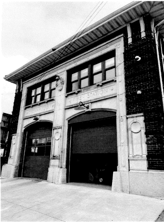
Building Front View (East side)
