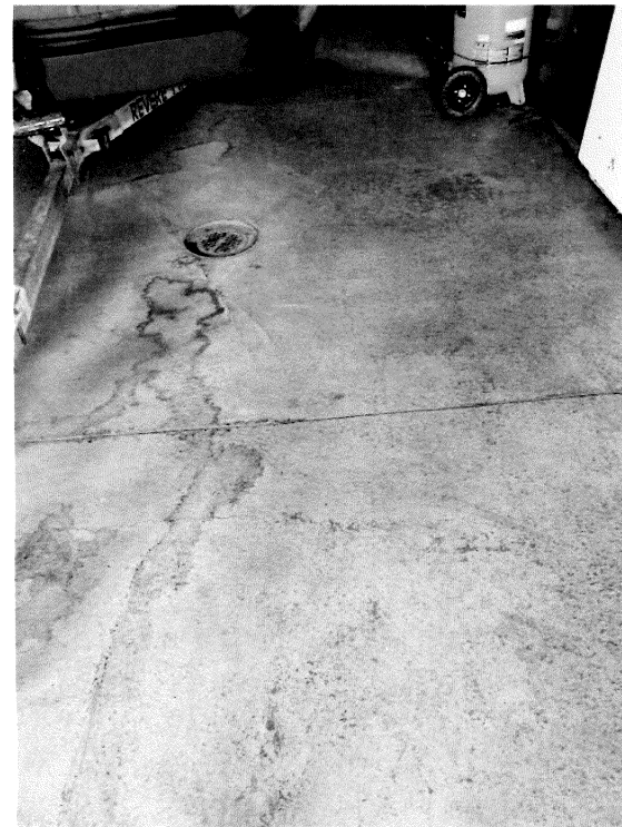
Floor Condition (Right Bay)
