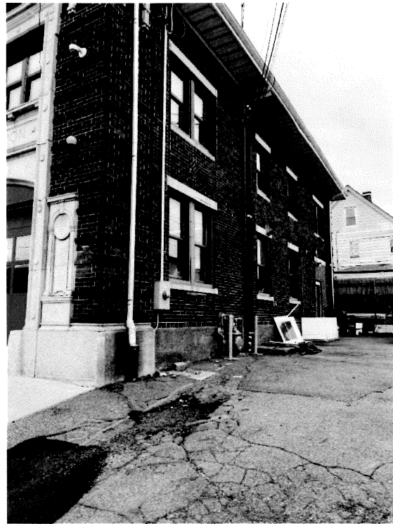
Building Side View (North side)
