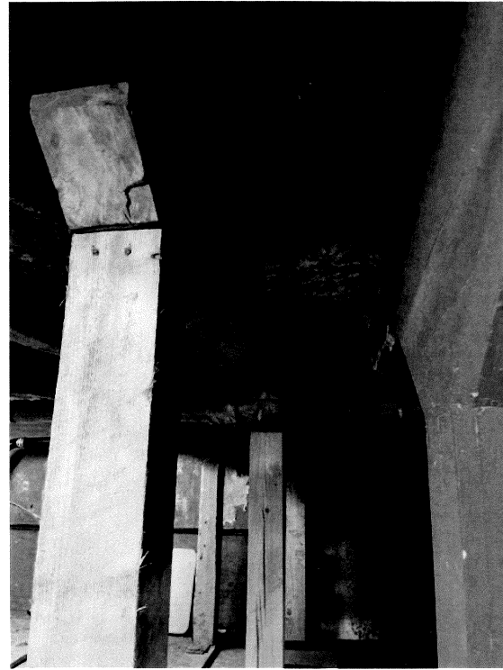
Floor Shoring (Left Bay)
